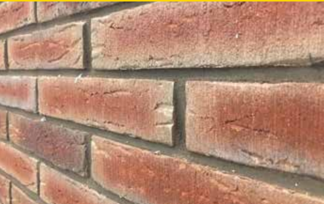
Panel bricks, splitting instead of sawing
